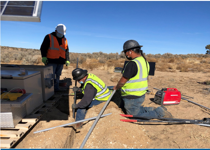
NTU Trainees laying the groundwork for a solar PV system.
